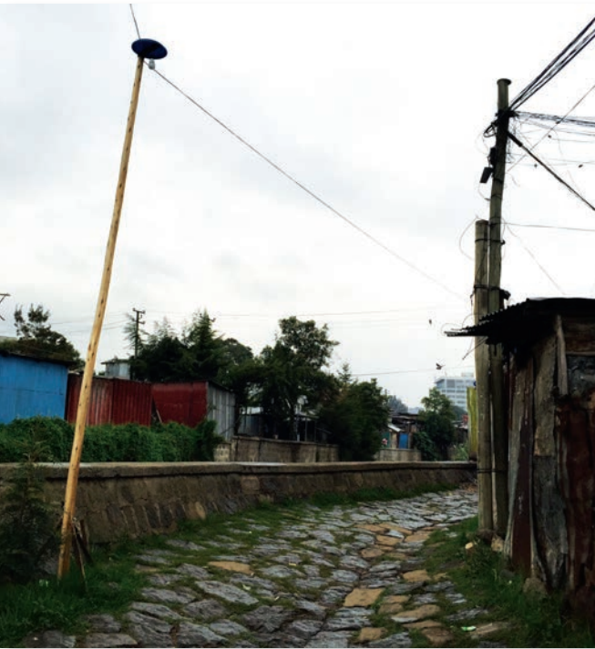
Electric lights and pole installed by community committee for security in WASH project, Addis Ababa.
